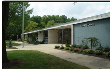
Frost 65 Frost Avenue 732-613-6852
